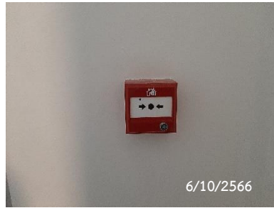
Fire Alarm Manual Station
